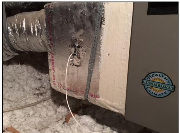
6. Install the Outlet Temperature Sensor. This sensor is installed after the heat exchanger. The sensor may be installed centered in the middle of the duct as shown. Use metal
