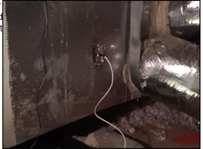
8. Connect the Outlet Temperature Sensor to the SYSTEM. The sensor connection has blue insulated wires. On an AC system -- the outlet temperature is cold.
