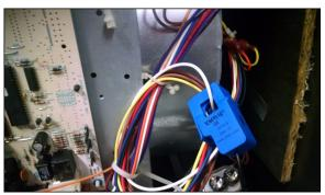
WARNING: If the SCT013 current probe jaws are not completely closed -- then the current measurement by the SYSTEM will be adversely affected. The SYSTEM will not operator and/or will operate inconsistently. Clamping the SCT013 current probe around both wires WILL give you a zero reading and the MCerberus® unit will not operate correctly.
